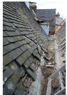
Above: one of the "tin hats" removed from the roof; below: the poor condition of one of the roof valleys
