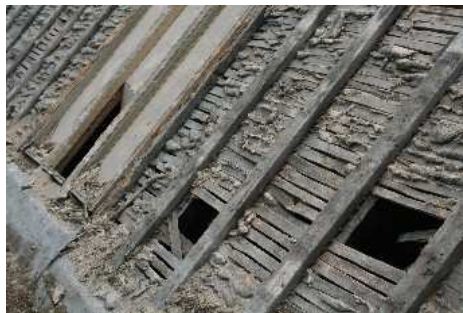
Left: Damaged wood battens visible where tiles have been removed. Right: inspecting the condition of the roof - note large gaps in tiles on the end gable
