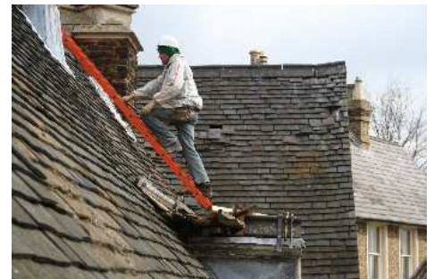
Left: Damaged wood battens visible where tiles have been removed. Right: inspecting the condition of the roof - note large gaps in tiles on the end gable
